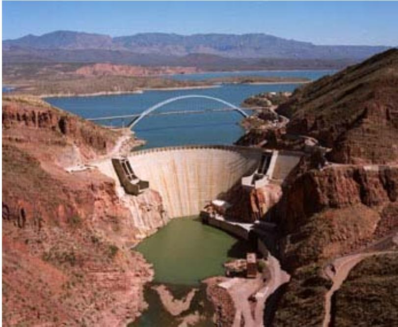
The shape of the arch may resemble a segment of a circle or an ellipse, and the arch may be curved in the vertical plane as well. Such dams are usually constructed of a series of thin vertical blocks that are keyed together; barriers to stop water from flowing are provided between blocks.
